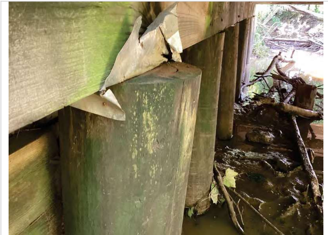
Abutment 2 pile A Alignment
