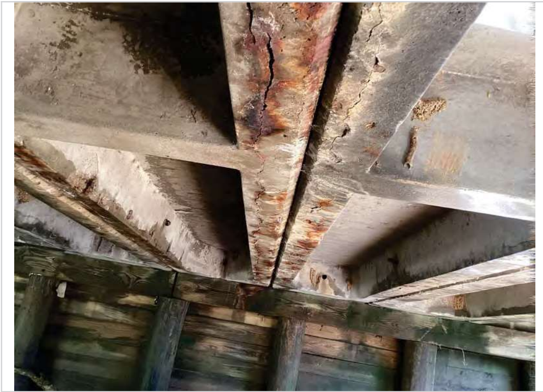
1/8" crack on slab E
