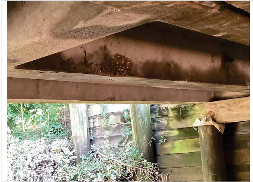
Spalling on slab B
