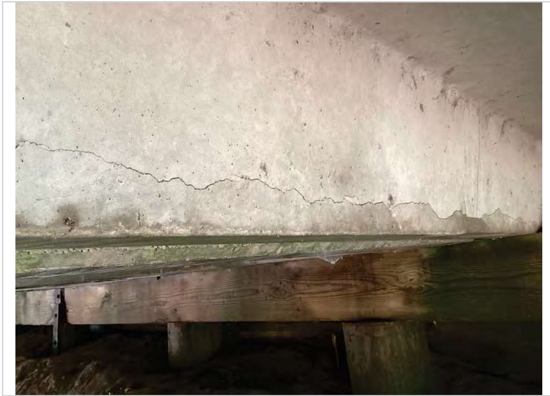
1/16" crack on slab A
