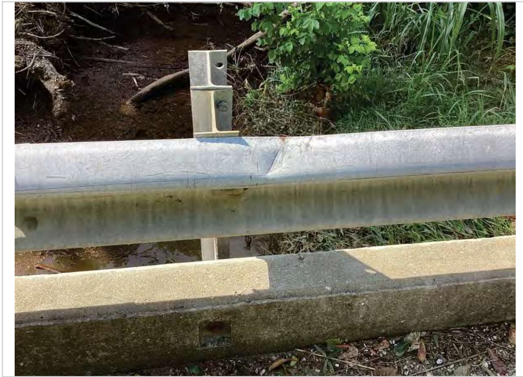
Right bridge rail damage
