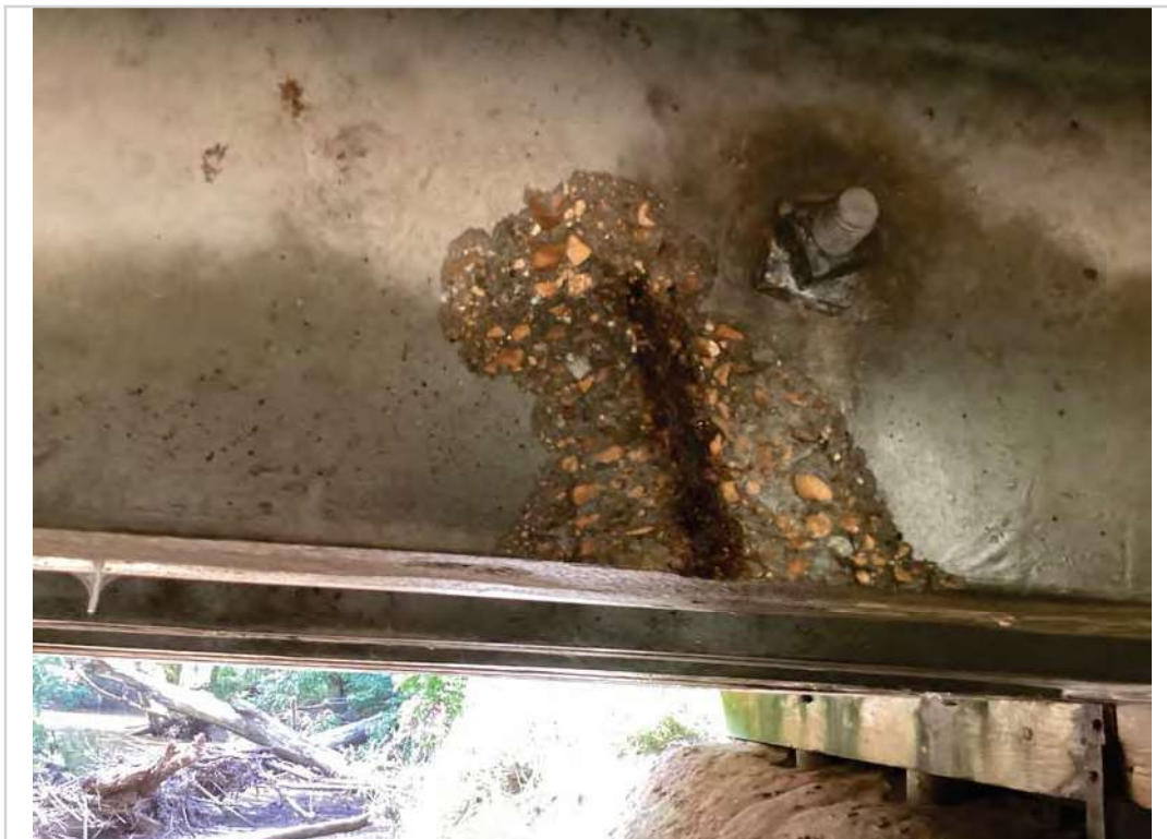
Spall to steel on slab B
