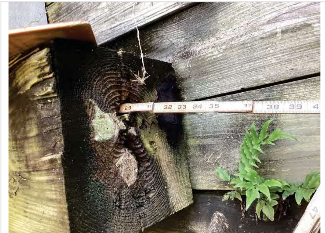
Right end of Abutment 2 cap decayed
