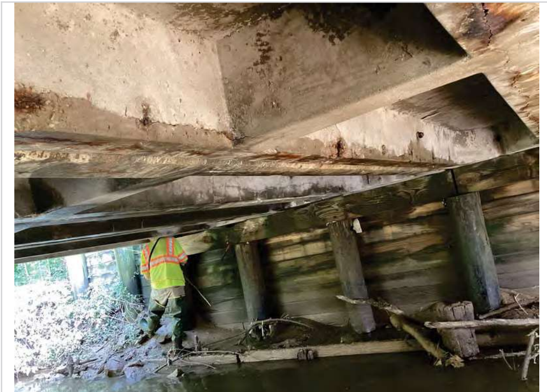
Impending spall on slab E
